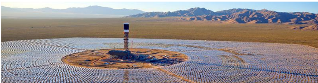
Aerial picture of the Ivanpah DSG Solar Power Facility in California
